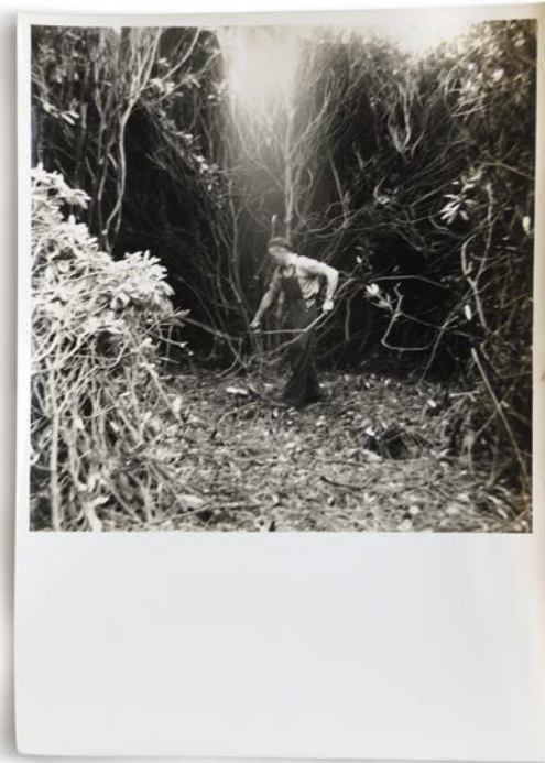
Workman cutting wood near the studio, photograph by Ivon Hitchens, 1950s.
